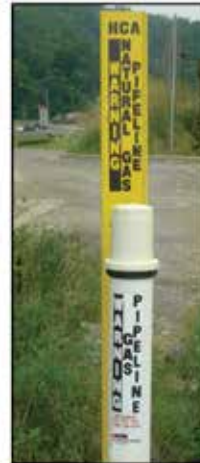
5. HCA marker and cathodic protection test station
