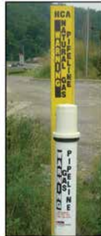
5. HCA marker and cathodic protection test station
